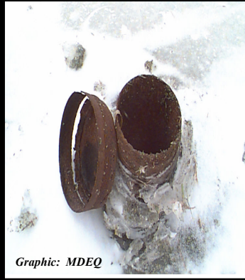
Abandoned Well in a Basement
