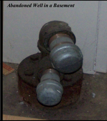
Abandoned Well in a Basement
